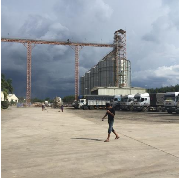
Figure 7: Storage tanks at the feedmill plant
