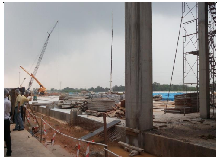
Figure 6: Phase 3 building under construction
