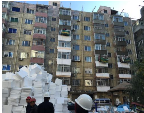
Figure 5. Polystyrene material used by GBT to be installed into existing buildings.
