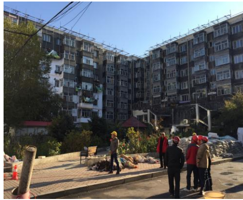
Figure 3. Walls are scrapped clean before the installation of polystyrene materials.
