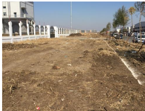
Figure 11. Fourth construction site that was visited.
