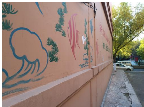
Figure 7. The Hebai estate project was completed in 2014, which is similar to the ongoing heat insulation project.
