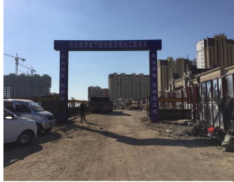
Figure 9. Second construction site that was visited.
