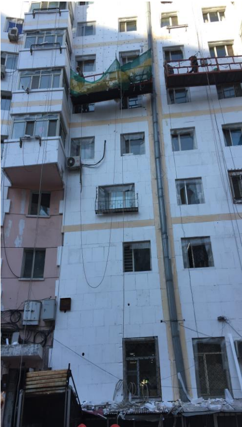
Figure 4. Polystyrene material used in existing building walls.
