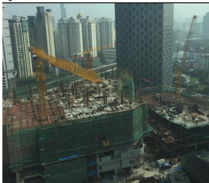
Figure 4: View of construction from Office Tower 3
